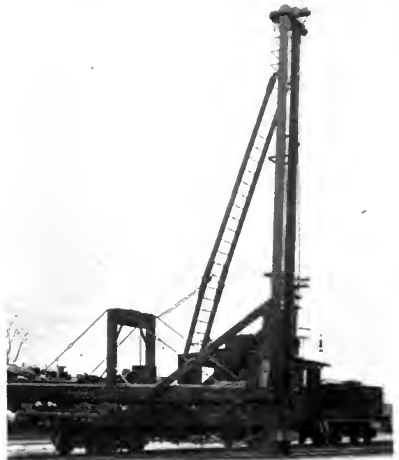
Self-propelling track layer for the C.O.R.C.C.
